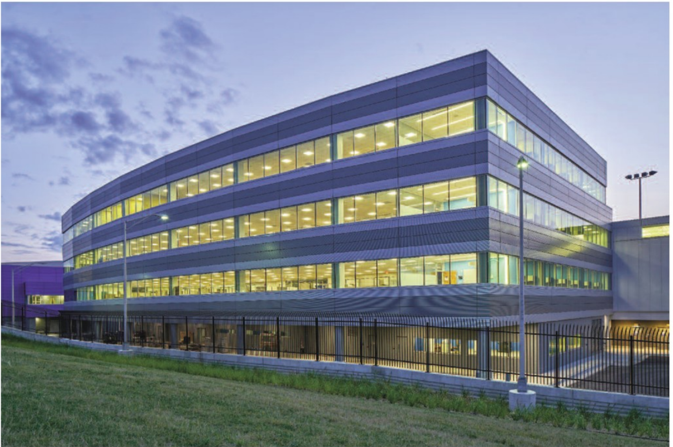
The exterior of the WCAA's Michael Berry Administration Building consists of a metal panel wall system, with ribbon windows skirting the perimeter. The design complements that of the North Terminal next door.
