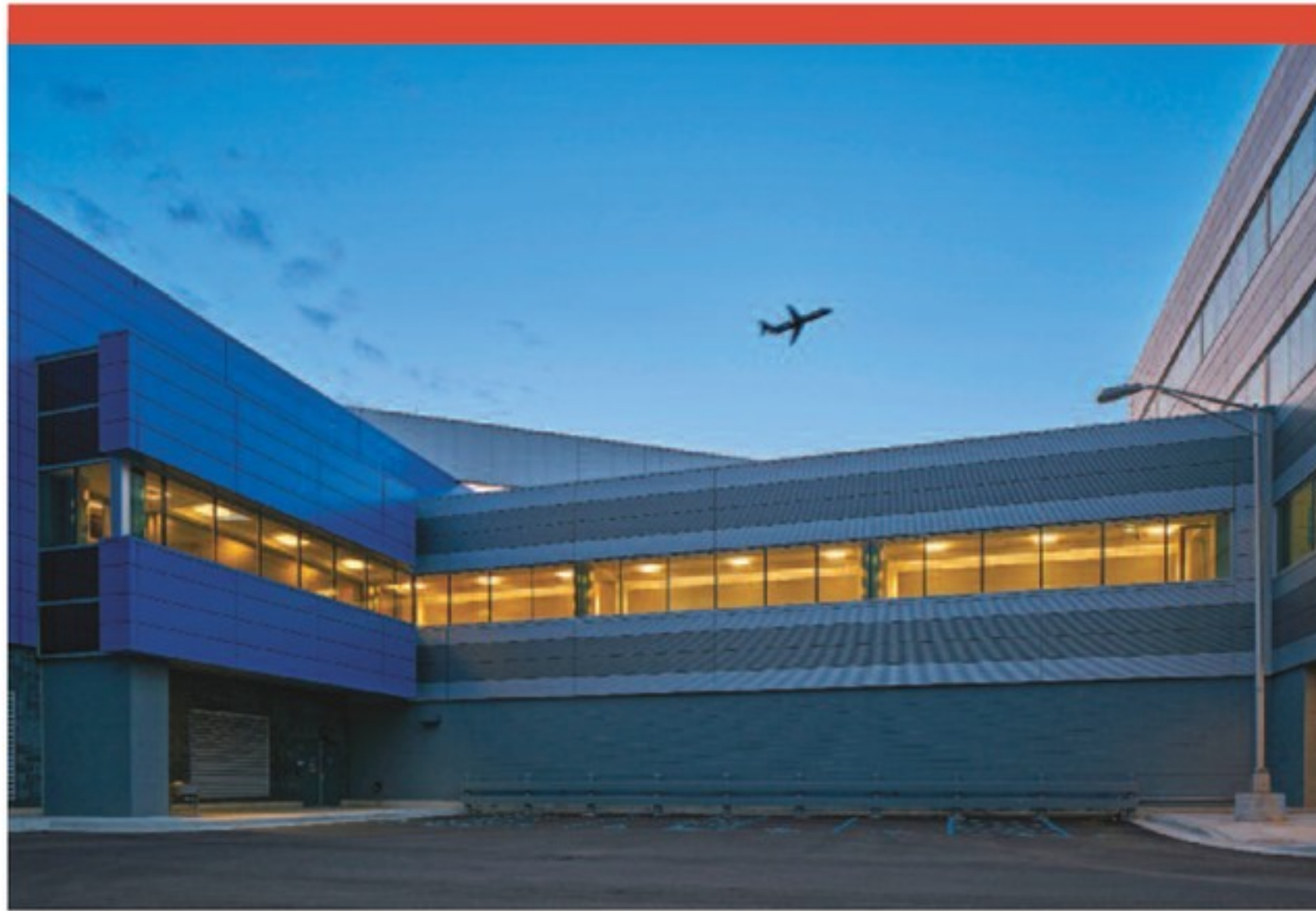
The public and employees enter the Berry building via an enclosed walkway bridge from the airport's North Terminal. At some points, the distance between the two buildings is as close as ten inches.
